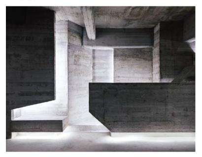
poured the concrete over them.' For Picault and Godefroy, adding more concrete to an existing basement seemed natural. Their method was used across the 600 sq m space, creating porous, jagged surfaces - the 'negative' of the sandbags structure illuminated with LED lights. Some of the walls' salient edges reach head height. 'That's als othe freedom of Mexico,' says Godefroy of the experimental and arguably hazardous design. 'It's not as restrictive in terms of regulations and safety measures'.
